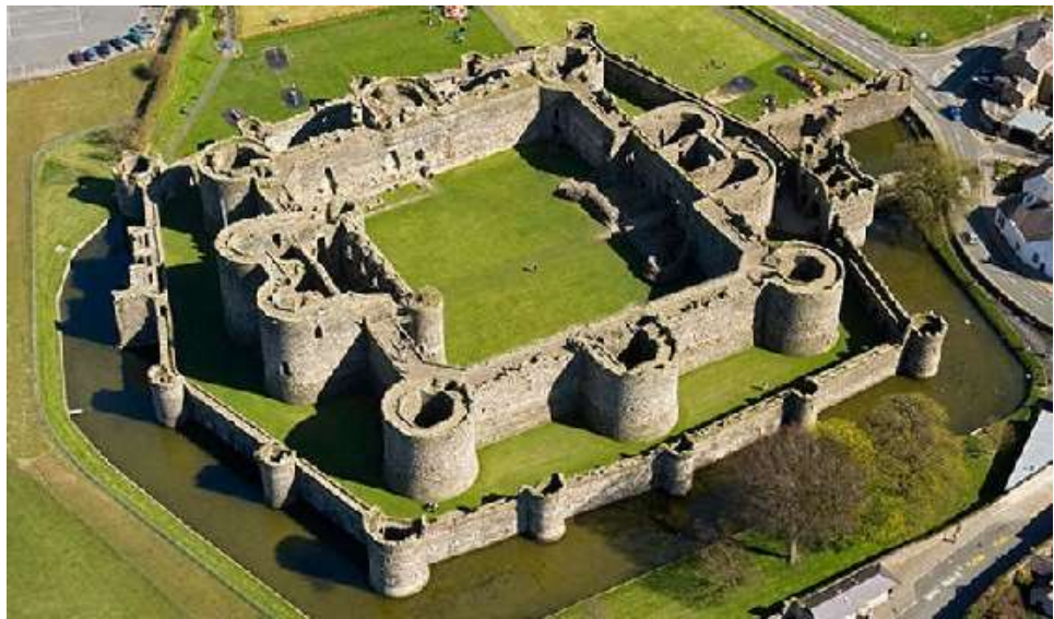
Figure 3 Curtain wall and towers at Beaumaris Castle
